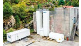
KNCC's demonstration facility (Cargo Tank Cylinders test rig)
